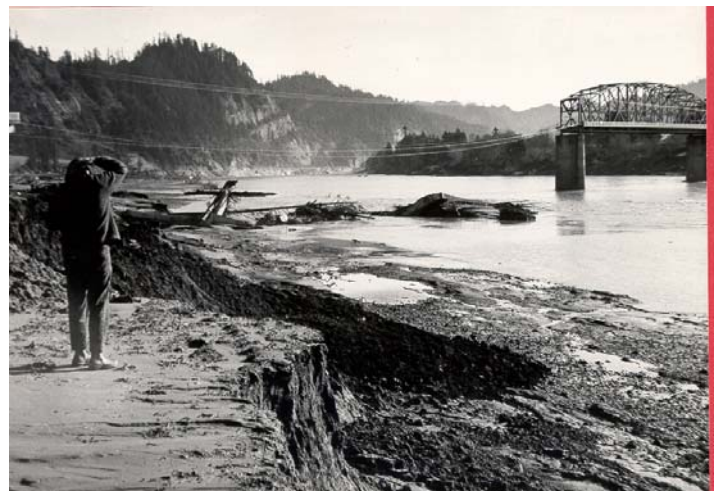
Figure 19 Eel River bridge north (downstream) of Scotia following the 1964 flood.
